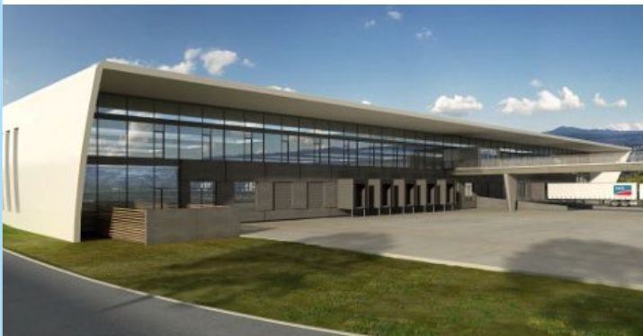
SMA Repair Center Niestetal
