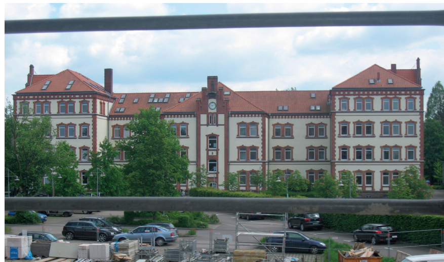
Existing Campus building A, former Prussian Cavalry barracks (Source: U. Schramm)
