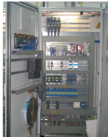
left: Atrium in the library right: Building automation system with 3000 sensors and actors (Source: U. Schramm)
