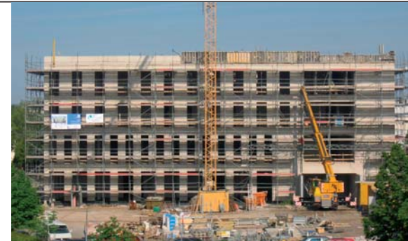
Construction site of new building, Minden Campus (Source: U. Schramm / May, 16, 2014)
