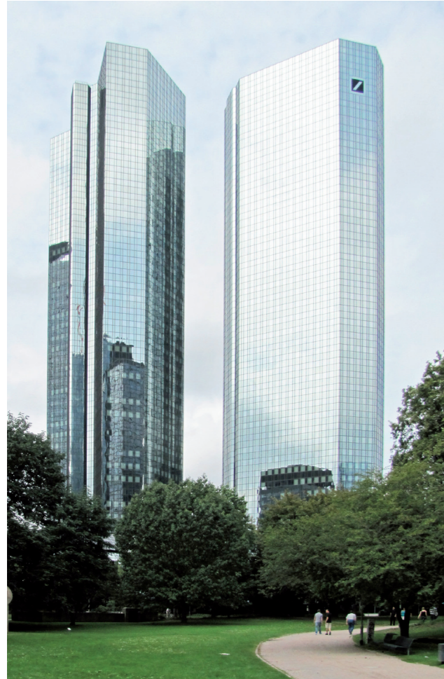
LEED-Platin/DGNB-Gold certified 02/2011 Deutsche Bank (renovation headquarters: Greentowers), Frankfurt am Main, Germany
